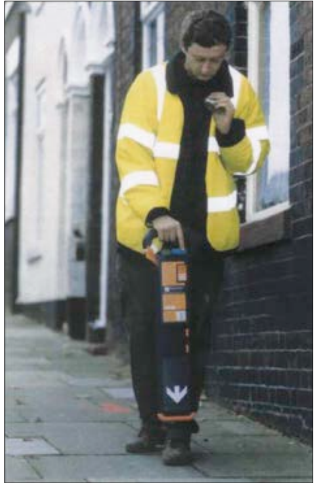
Figure 5 Using a cable locator
