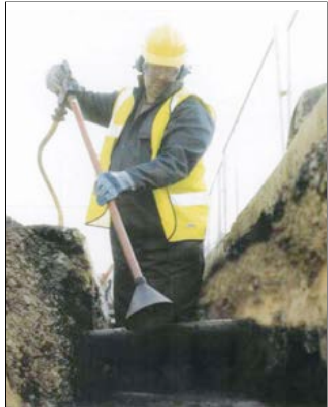
Figure 7 Using an air digging tool
